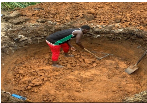
Manual excavation of the digester pit
