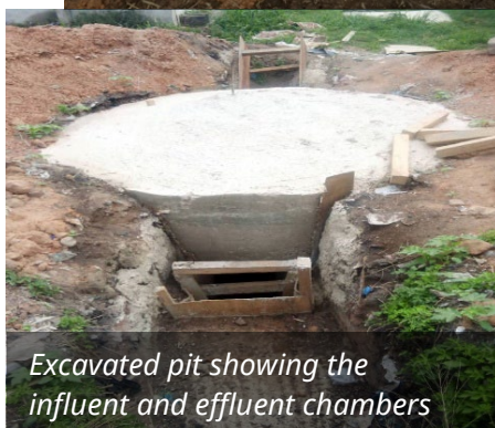
Manual excavation of the digester pit
